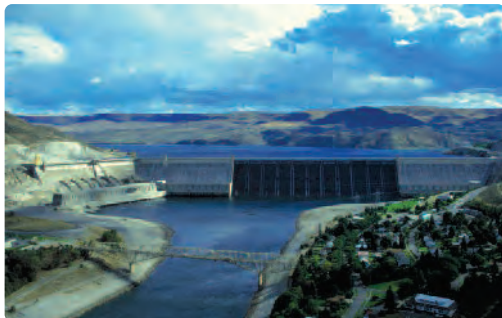
The Grand Coulee Dam
